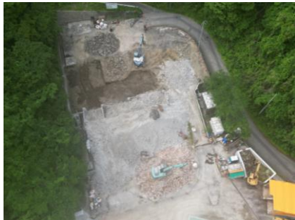
〔ごみ焼却炉・炉室解体状況〕
